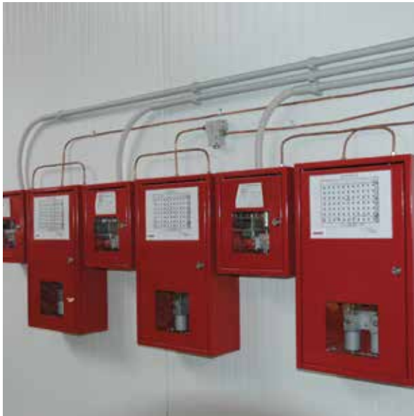
Fig. 1 Example of pneumatic smoke exhaust control system
