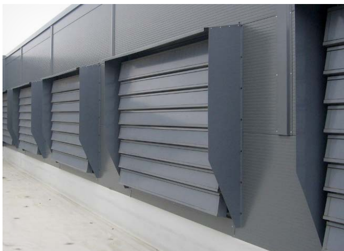
Photo. III–IV Façade mounted mcr LAM vents equipped in rain shields
