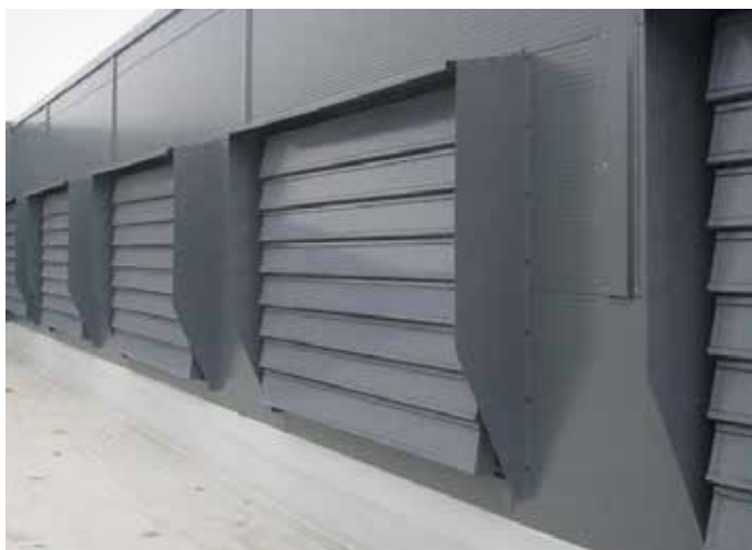
Zdjęcie. III-IV Façade mounted mcr LAM vents equipped in rain shields
