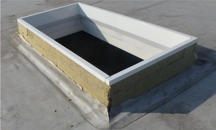
Fig. 31. Insulated base (insulation thickness 50 mm).
