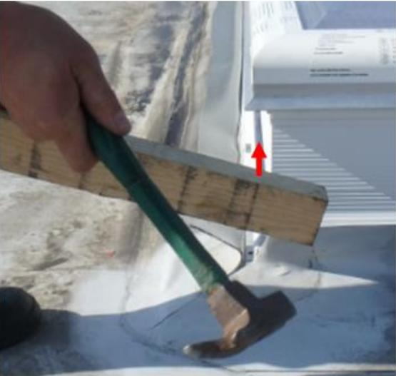
Fig. 42. Hammering the connector.
