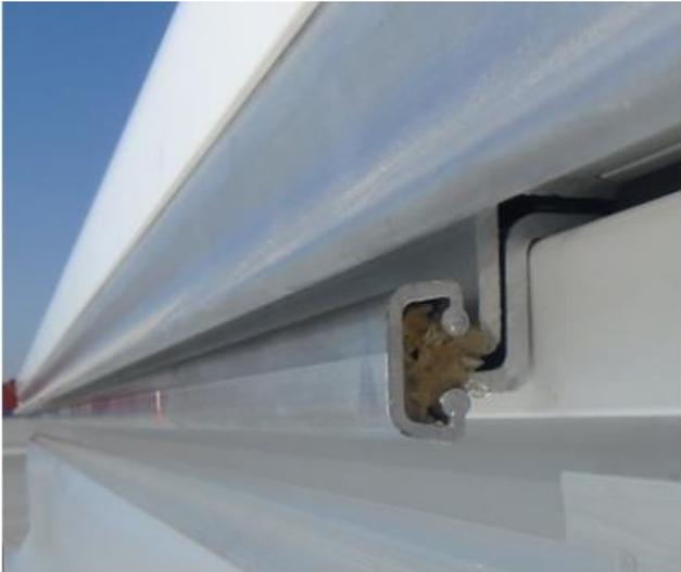
Fig. 43. Hinge connection mounted.
