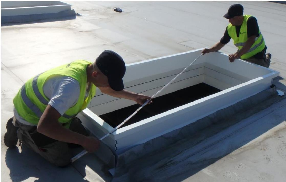
*Fig. 29. Checking diagonals.*
