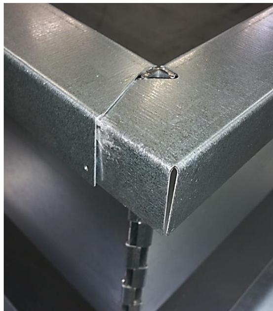
*Fig. 25. Properly connected walls.*
