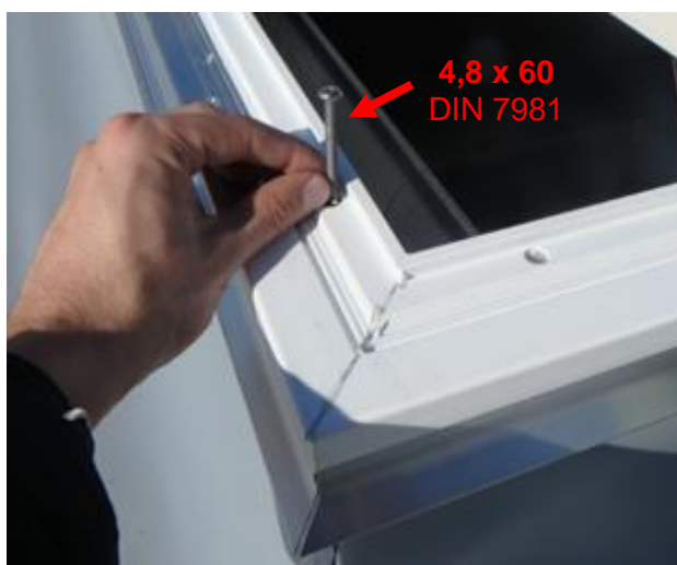
Fig. 35. Screwing the PVC top flange of base to the metal base.
