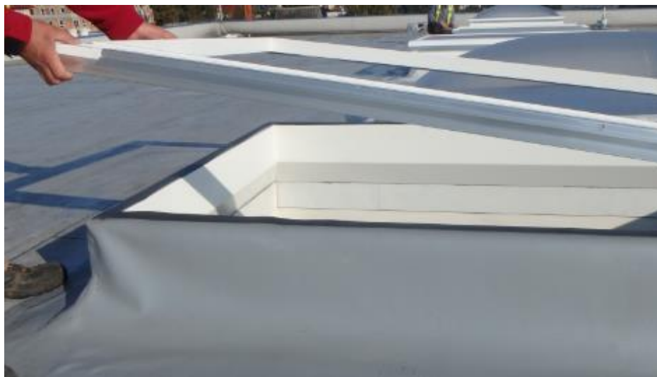
Fig. 34. Putting PVC top flange of base on the PES gasket.
