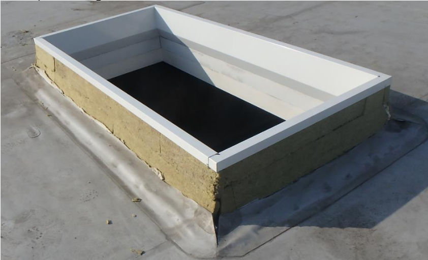
Fig. 31. Insulated base (insulation thickness 50 mm).
