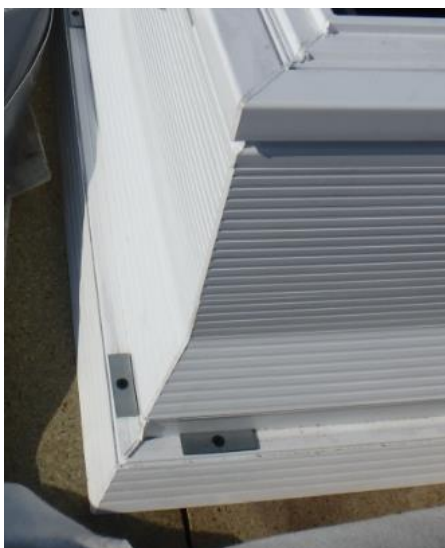
Fig. 16. Fixing the PVC base to the roof
