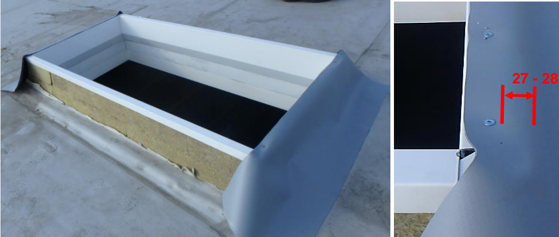
Fig. 32. The membrane is rolled up on the base and fixed with screws. Note the location of the screws.
