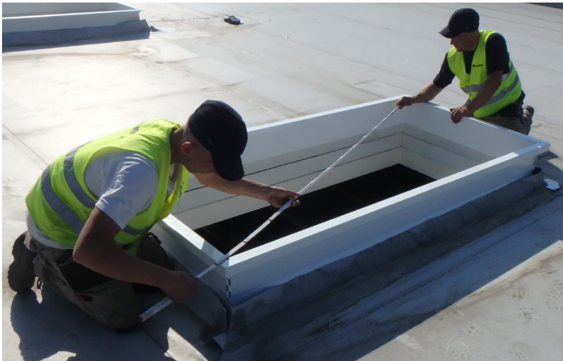
Fig. 29. Checking diagonals.
