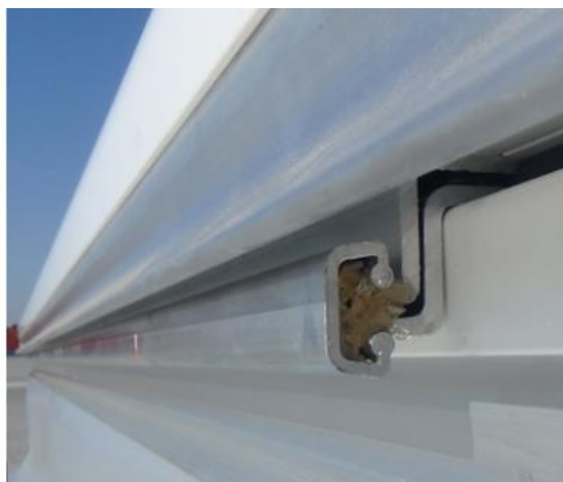
Fig. 43. Hinge connection mounted.
