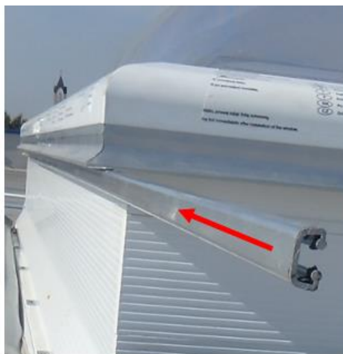
Fig. 41. Sliding the connector on.
