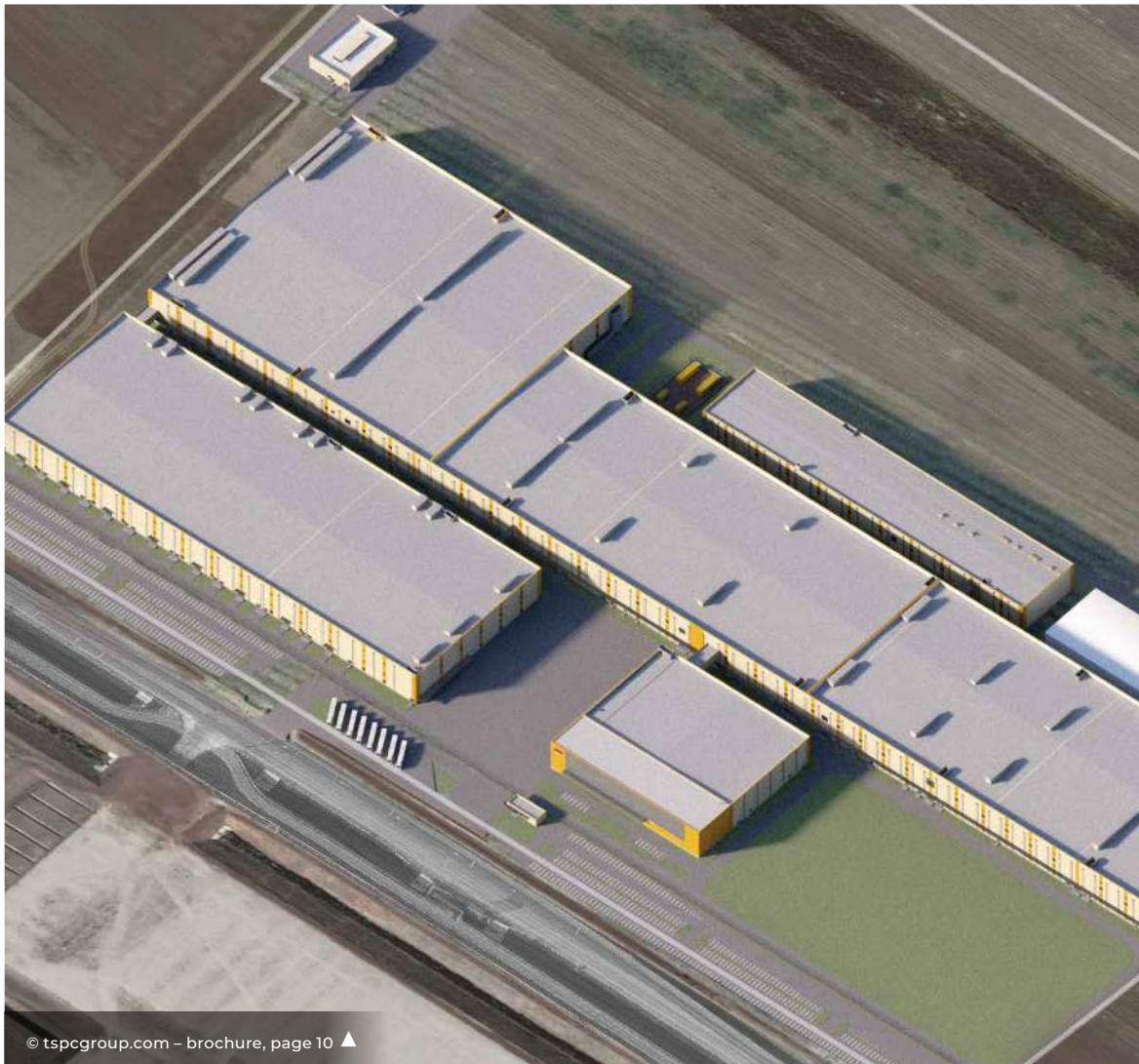
“Eve Power” battery production plant (Debrecen, Hungary)
