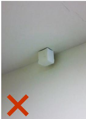
7. mcr ICS Pro pressure transmitters should be installed with the connection stubs of the pneumatic system facing downwards, which prevents the penetration of dust resulting from work carried out on site. The drawing below indicates the site where dust penetrates due to incorrect installation with the connection stubs facing upwards, which will eventually result in incorrect parameter readings due to the accumulation of dust.
