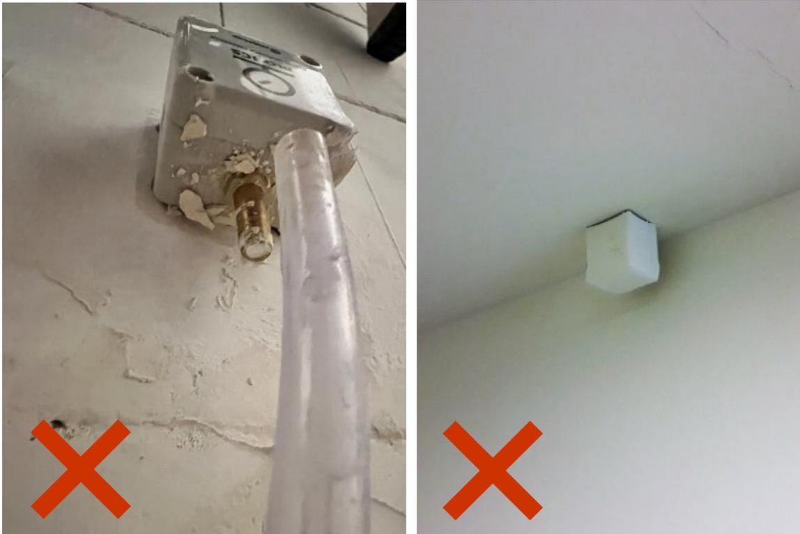
7. mcr ICS Pro pressure transmitters should be installed with the connection stubs of the pneumatic system facing downwards, which prevents the penetration of dust resulting from work carried out on site. The drawing below indicates the site where dust penetrates due to incorrect installation with the connection stubs facing upwards, which will eventually result in incorrect parameter readings due to the accumulation of dust.
