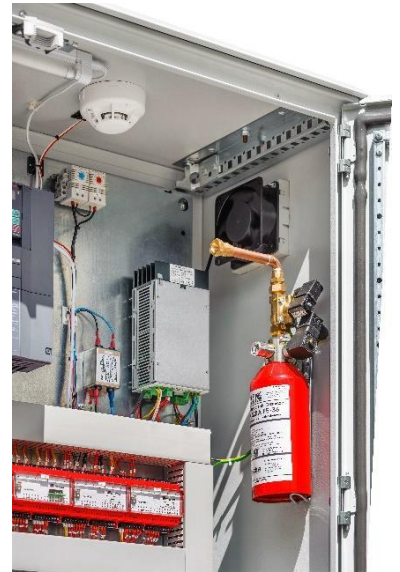
Fig. 12. FFES inside the panel.
