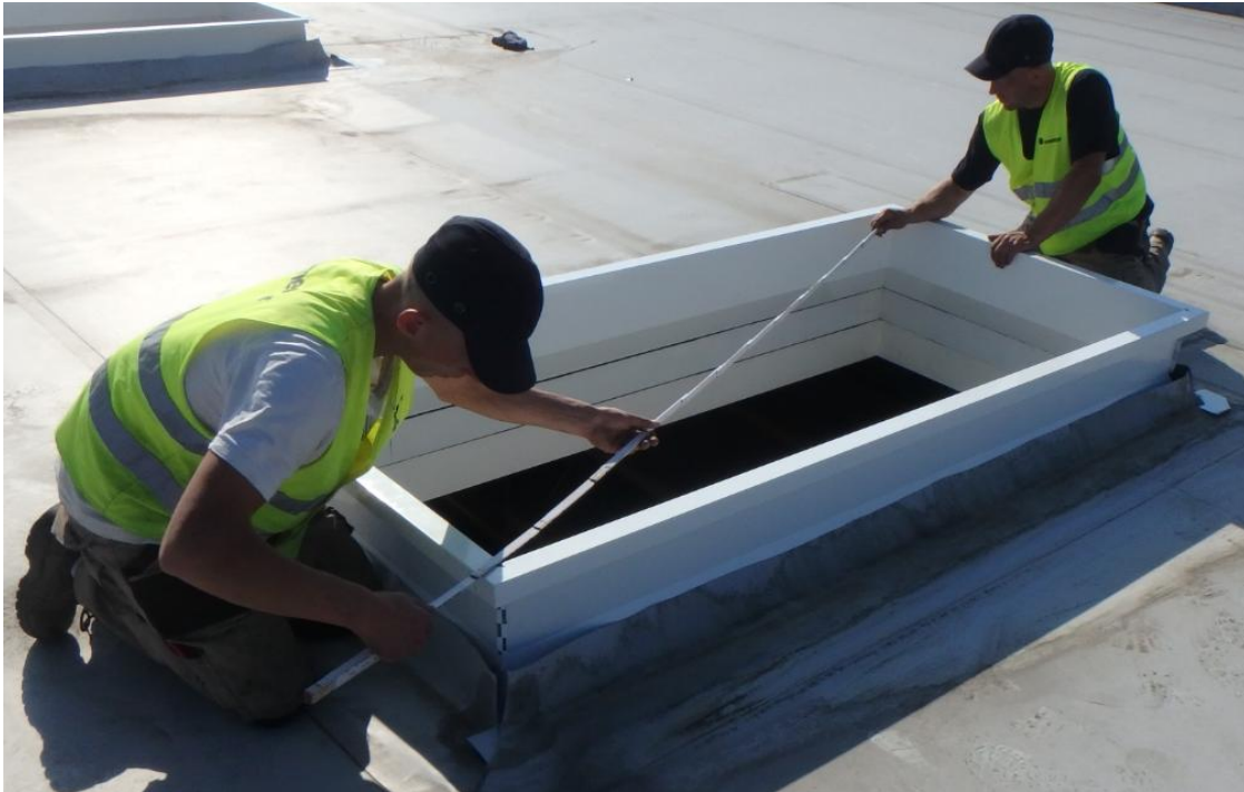
Fig. 29. Checking diagonals.
