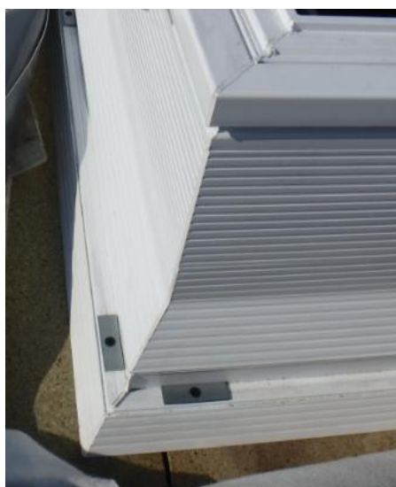
Fig. 16. Fixing the PVC base to the roof
