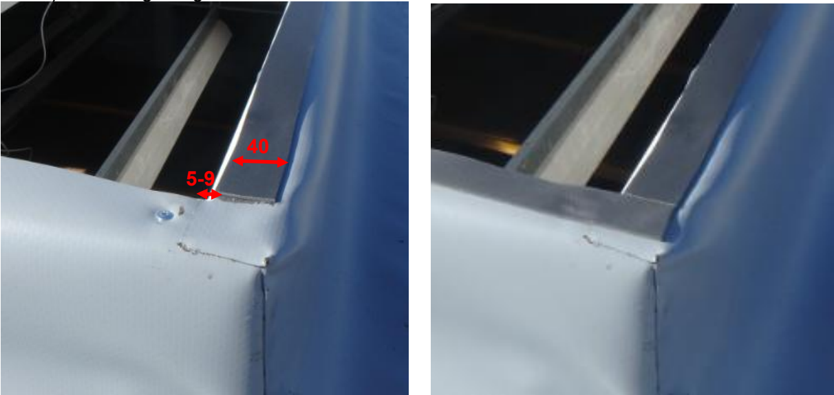
Fig. 33. Attached gasket PES 40x3. Pay attention to the butt joint of the gasket in the corner.
