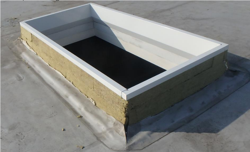
Fig. 31. Insulated base (insulation thickness 50 mm).
