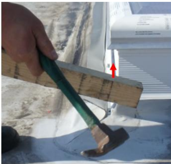
Fig. 42. Hammering the connector.
