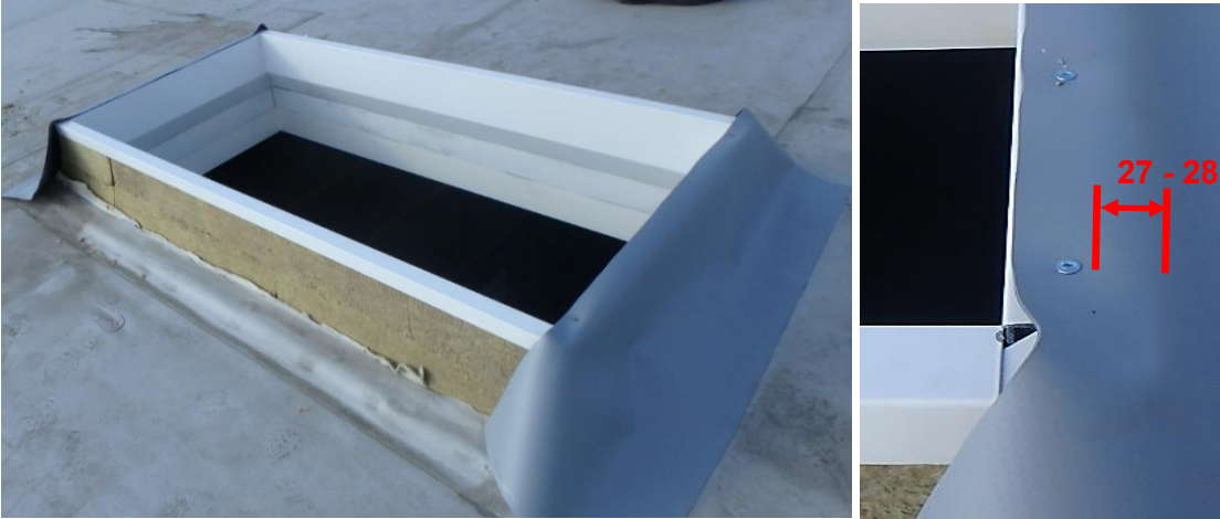
Fig. 32. The membrane is rolled up on the base and fixed with screws. Note the location of the screws.
