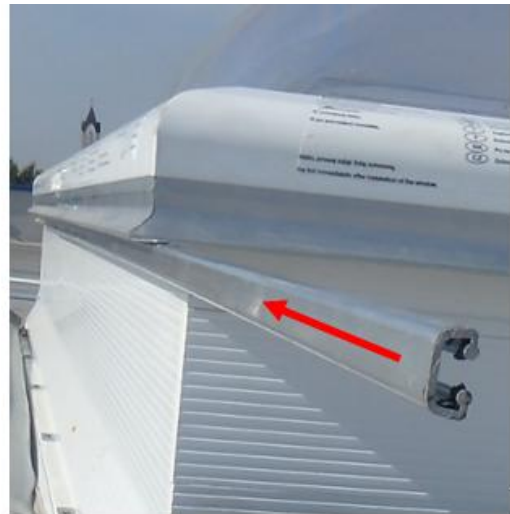
Fig. 41. Sliding the connector on.
