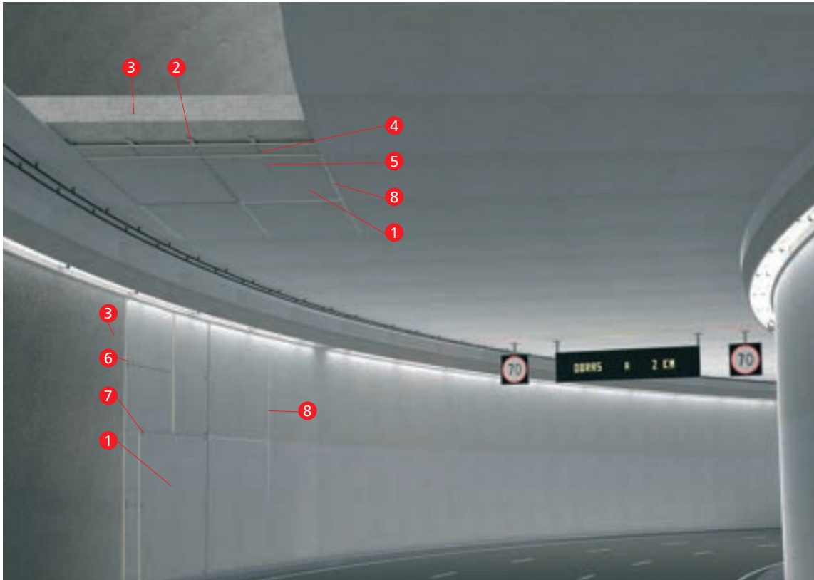
» Horizontal view of the ceiling
