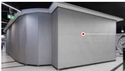
separated area: non-standard shape of the curtain with corner connections
